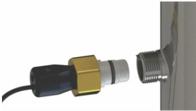
Figure 6. UV Sensor Installation
